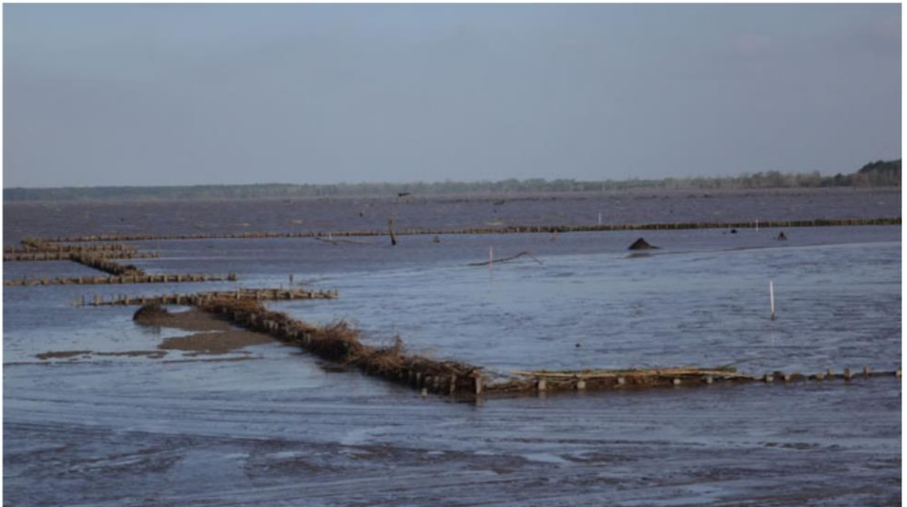
Suriname is aiming to reverse coastal erosion of mangroves countering destructive erosion along the country's coastline with these permeable dams breaking the waves and trapping sediment and reclaiming land. Credit: Sieuwnath Naipal
